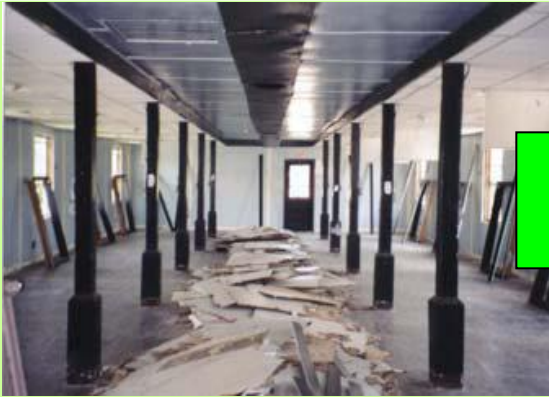
1. 拆除門窗及室內裝潢
